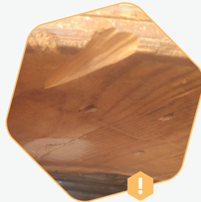
REPAIR THE DRUM
