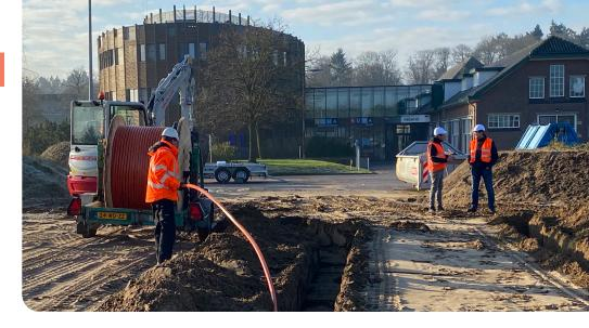
FuturePath® ECO has also been tested and proven in the field. Dura-Line's team facilitated a successful field trial conducted by Amadys and various contractors in the Netherlands, which confirmed equivalent performance to regular MicroDuct products, including during duct laying and cable jetting.
