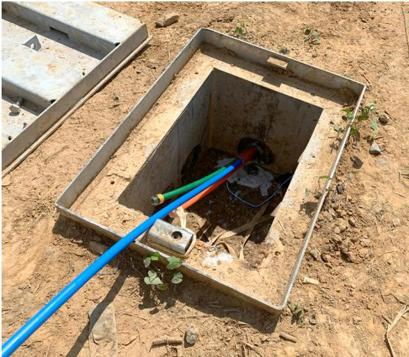
placement of the MicroDuct 16/12 mm with a Condux Gulfstream, and successfully jettied the MicroDuct into the existing 2-inch PVC in a similar method to what would occur in a MicroDuct override. Placement of a 24-count, 7.6mm OD micro fiber optic cable followed with a Plumettaz MiniJet.
